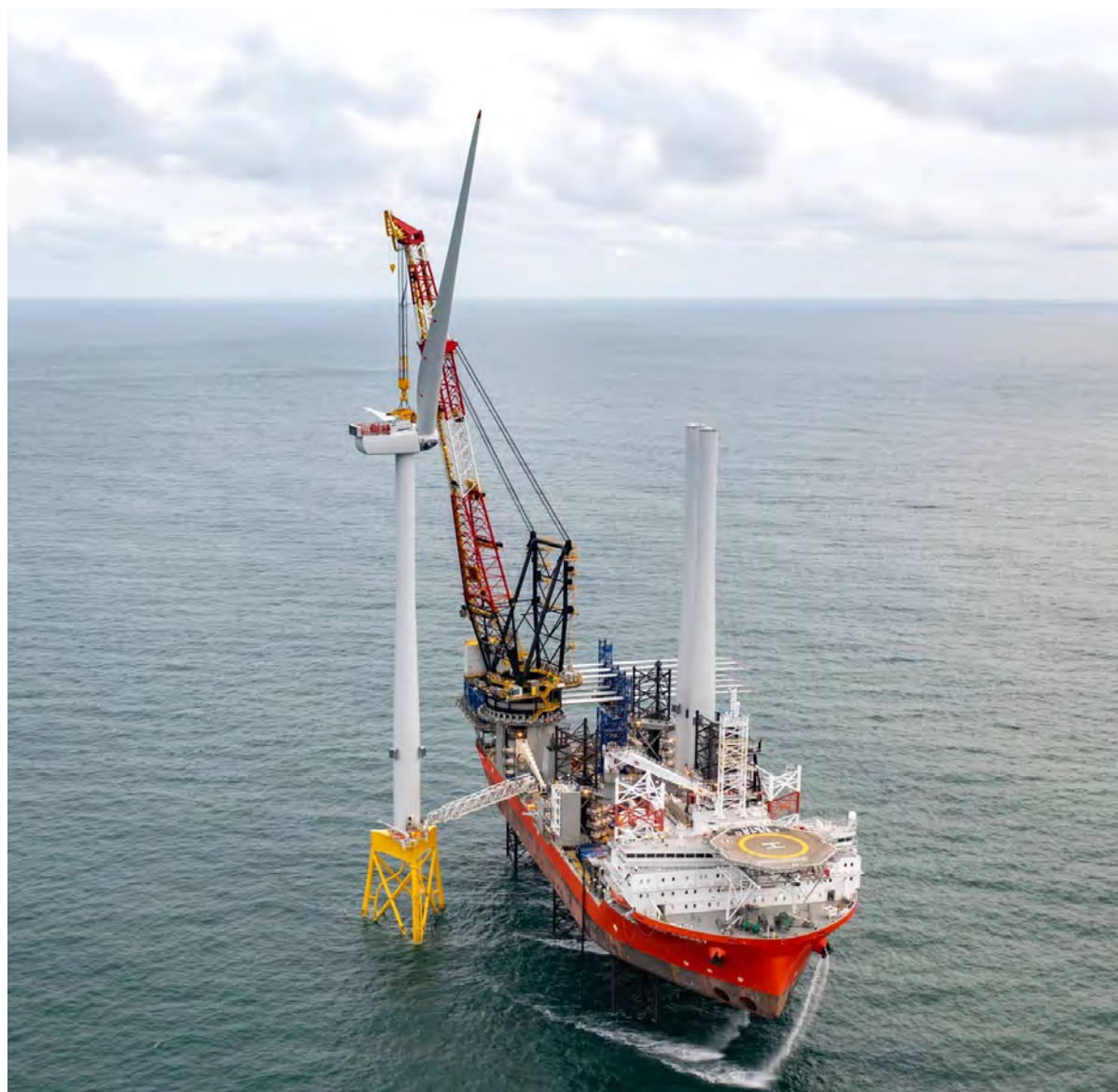
Seagreen Offshore Wind Farm Turbine Installation
