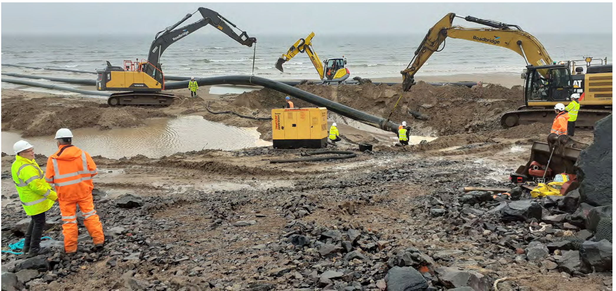
Seagreen 1 Landfall Cable Installation Works at Carnoustie
