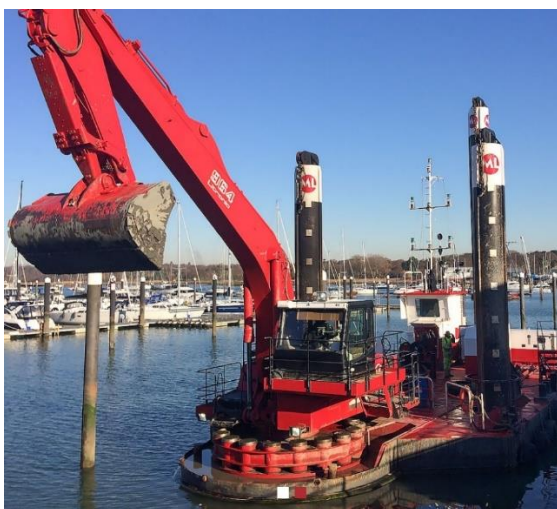
Figure 2.5 Offshore Backhoe Excavator
