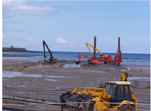
Figure 2.1 Open Cut Trenching
